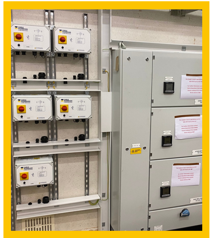
CableGuardian System Installation, Network Rail, Wales and Western
