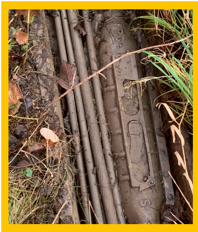
Faulty Cable Joint
